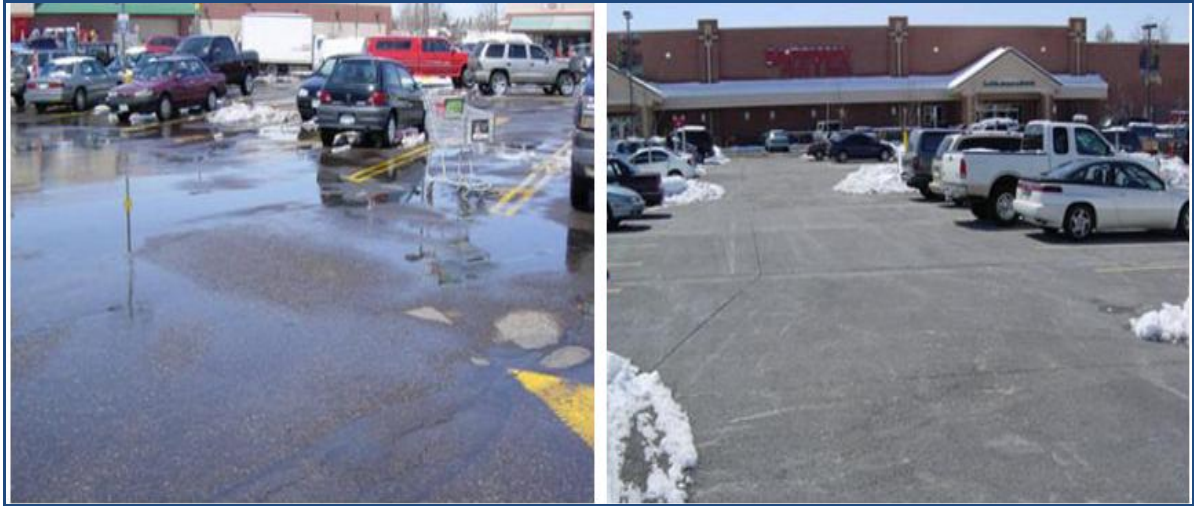
Figure 2-1. Conventional Asphalt Concrete Pavement and Pervious Concrete Pavement after Snowstorm (Adopted from [24])
